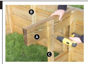
Position Leg Brace C 350mm (nom.) from base of Leqs B and attach using 4no. 70mm Screws - 2no. per Leg A (Fig.2). Repeat procedure for remaining Leg Brace C.
