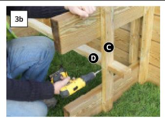
Position Central Brace D as shown in Fig.3a and attach to Leg Braces C using 2no 70mm Screws – 1no per Leg Brace C (Fig.3b).
