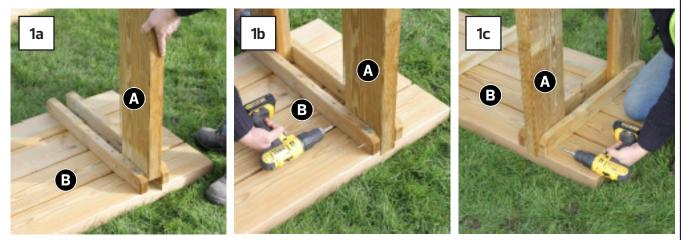
Position Leg A as shown in Fig.1a and attach to Table Top B using 4no 70mm Screws - 2no per side (Figs.1b & 1c). Ensure Leg A is completely flush into groove before fixing. Repeat procedure for remaining Legs A.
