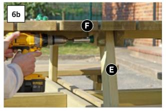
Assemble the The table top. locate holes and insert the four 130mm Bolts, and attatch the Plastic Nut Covers, 20mm Washers and Nuts. then fully tighten all fixings.
