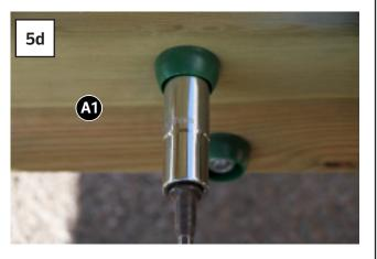
Attach Nut Cover Base (Fig 5c), 20mm washers and nuts. Do not fully tighten at this stage. Repeat for remaining three Table-Top Supports.
