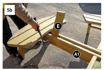
Insert Table-Top Support (E), align bolt holes and insert two 130mm bolts (Fig 5a & 5b).
