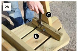
Position Leq (C) as shown in Fig 2a, align bolt holes and insert two 90 mm bolts & attach 30mm washers, spring washers and nuts (Fig 2b). Do not fully tighten at this stage. Repeat process for the remaining 7 legs.
