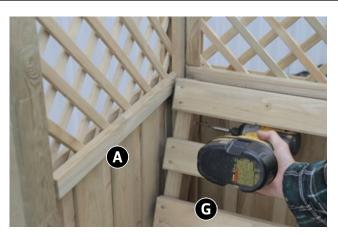
Place Seat Back Assembly (G) onto fixed section of Lid/Seat Assembly (F) and fix in position using 4 x 60mm screws (2 x Screws per side).
