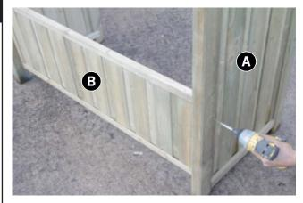
Place Front Panel B between battens on Side Panels (A) (flush with outer edge of battens) and fix through Side Panels (A) using 4 x 60mm screws (2 x Screws per side).
