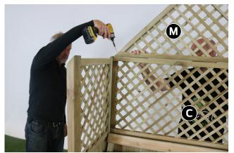
Fix Triangular Trellis Panel (M) to Rectangular Trellis Panel (C) using 2 x 60mm Screws.
