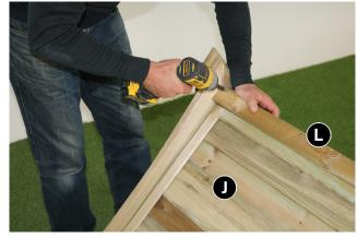
Join 2 x Roof Capping's (L) using 3 x 40mm Screws and attach to Roof Panels (J) using 4 x 40mm Screws (2 x Screws per end).
