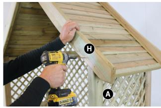
Place roof assembly on to Side Panels (A) and Triangular Trellis Panel (M). Fix in position through Fascia's (H), into Side Panels (A) using 4 x 60mm Screws. (1x Screw per Fascia (K)).
