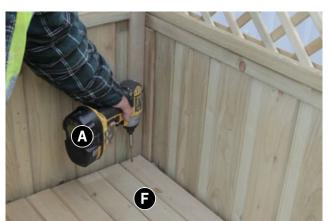
Position Lid/Seat Assembly (F) (lipped lid edge to front) onto upper battens of side panels and fix as shown using 4 x 60mm screws (2 x Screws per side).
