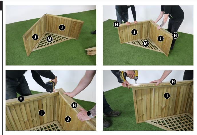
Using Triangular Trellis Panel (M) as a guide, set out Roof Panels (J) and 2 x Fascia's (H) as shown. Note: Ensure roof board overlaps are in correct orientation as to avoid rainwater ingress.
