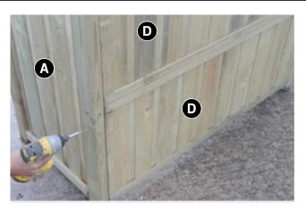
Place 1x Back Panel (D) directly beneath Rectangular Trellis Panel (C) and fix through posts using 4 x 60mm screws (2 x Screws per side). Place remaining Back Panel (D) beneath fixed Back Panel (D) and attach through posts using 4 x 60mm screws (2 x Screws per side).
